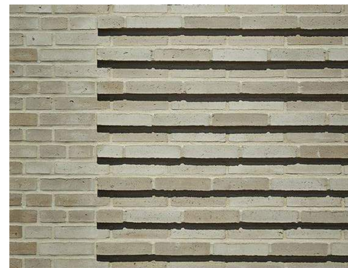
HORIZONTAL BRICK REVEAL DETAILING
