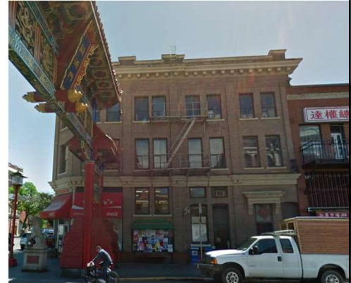
North Façade along Fisgard St.
