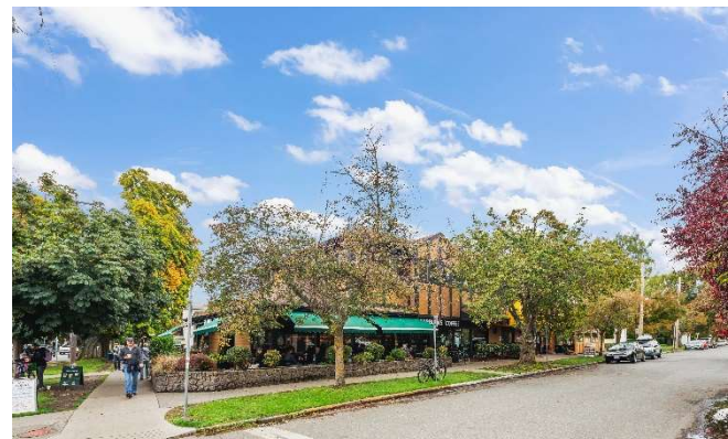
Figure 2 - Existing Building Pendergast Street
