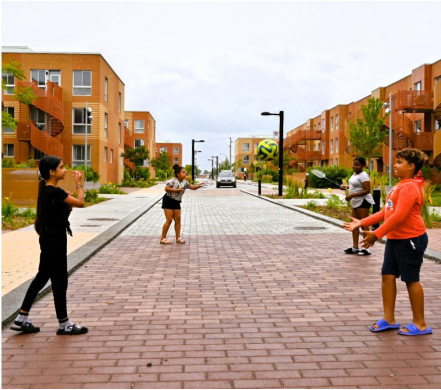
Family-friendly sites and buildings: Built form and shared-traffic laneway in an affordable housing development in Montreal [SBT Architectes and Vlan Paysages - Habitations Saint-Michel-Nord; Image credit: Vlan Paysages]
