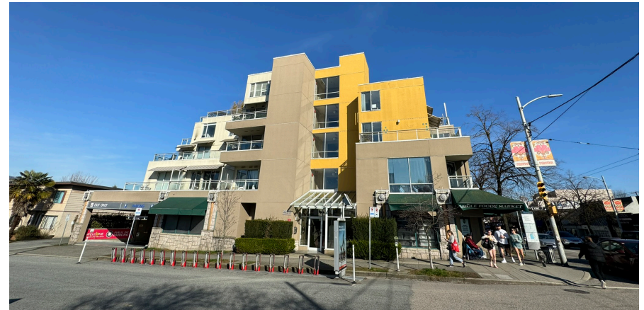
Daylight access to elevator lobbies and corridors expressed on the exterior of a family-friendly mixed-use development in Vancouver [HBBH - 1978 Vine Street (Capers Building); Image credit: City Staff]
