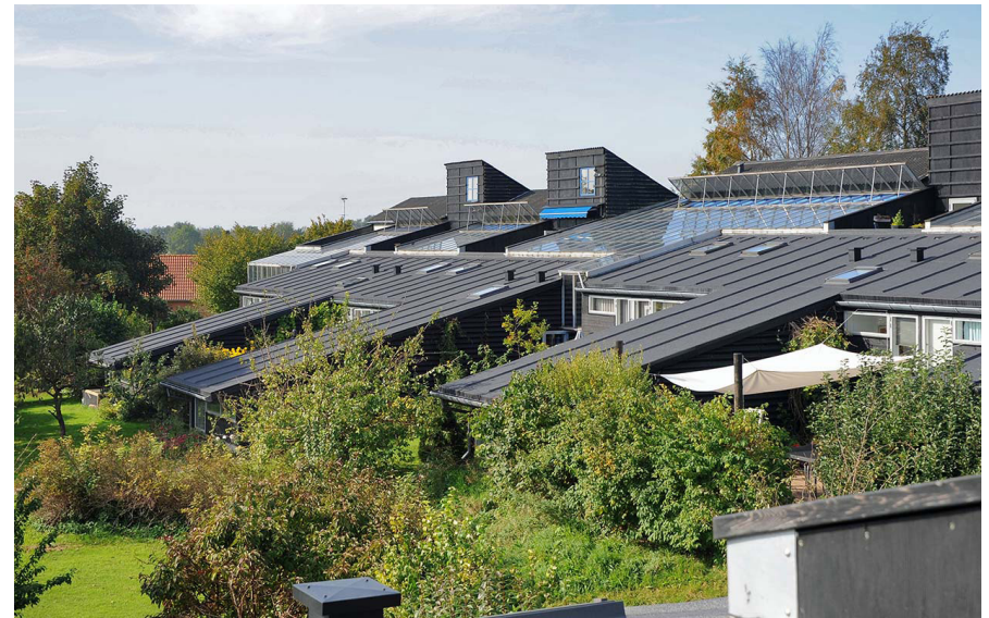
Skylights and roof monitors enable these dual-aspect family-friendly townhomes that are otherwise flanking a central community atrium [Vandkunsten - Savverket Cohousing; Image credit: Vandkunsten]
