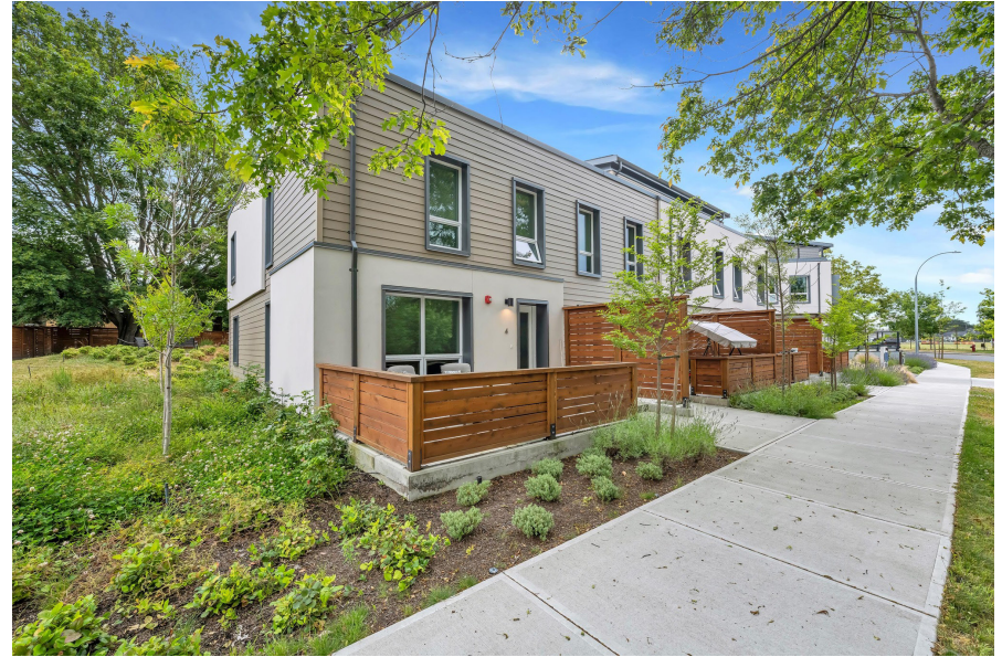
Family-friendly townhomes and their private patios with privacy fences and strategically located deciduous trees for seasonal shading in Saanich [HCMA Architecture + Design - Townley Place Affordable Housing; Image credit: H&R Exterior Finish]
