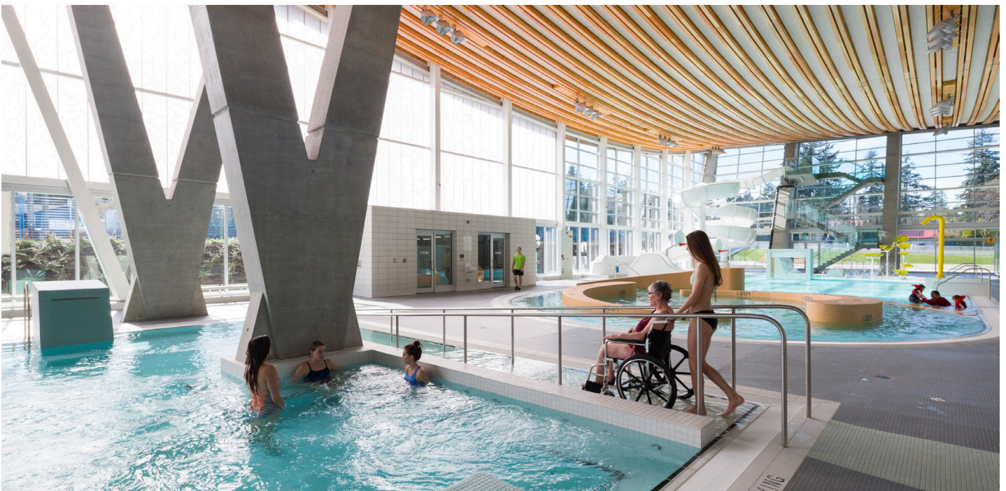
Grandview Heights Aquatic Centre, sloping floor pool access
