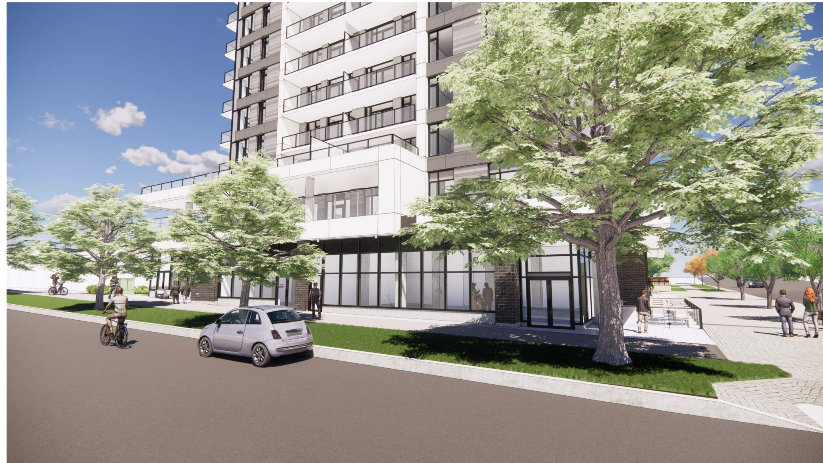
VIEW OF 12 STOREY TOWER FROM COOK STREET
