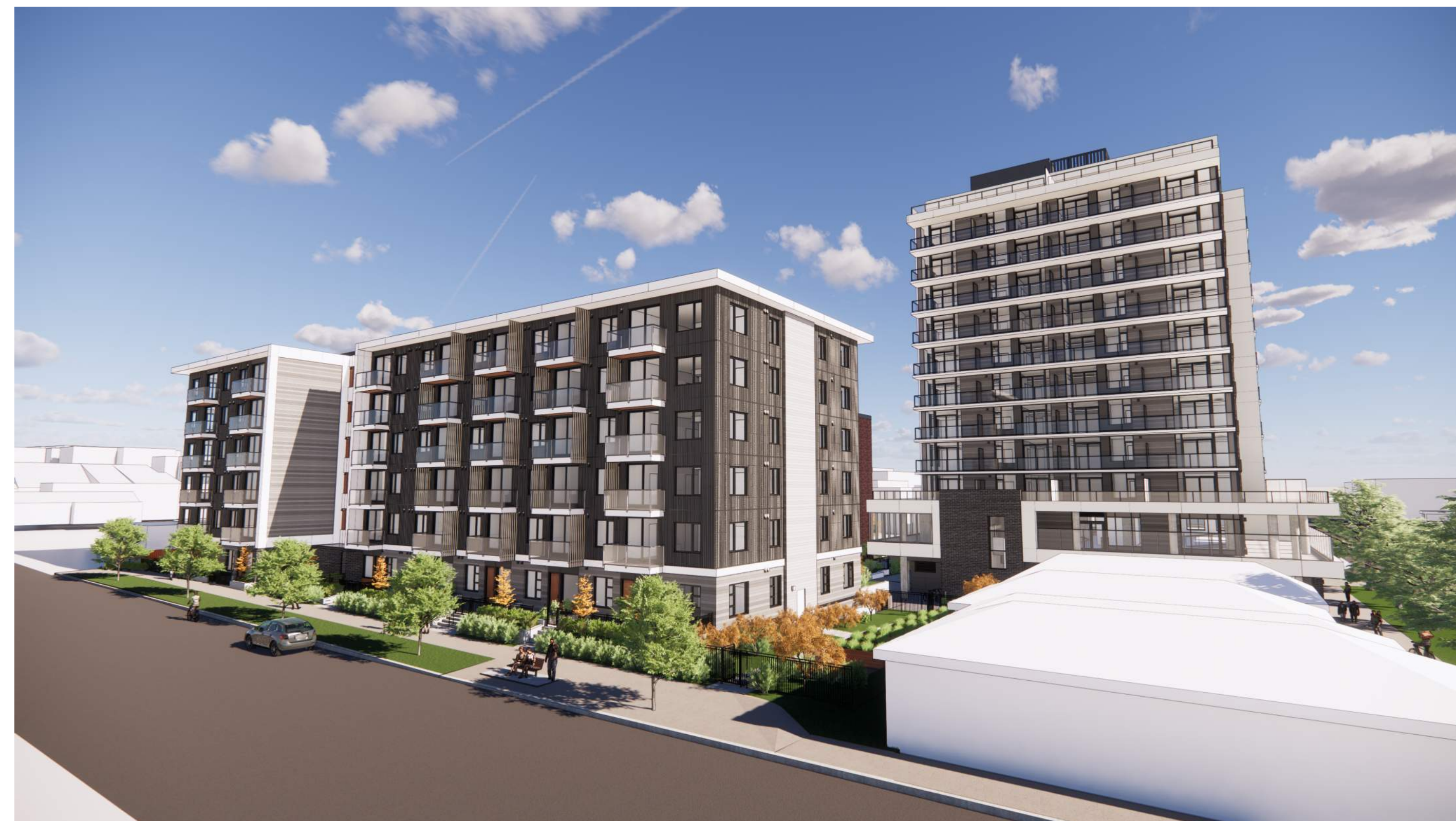
VIEW LOOKING EAST ALONG JOHNSON ST
