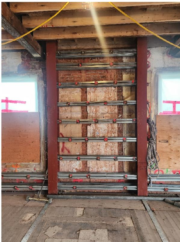
**Figure 5 – Back of Second Storey Retained Brick Wall along Hillside**
