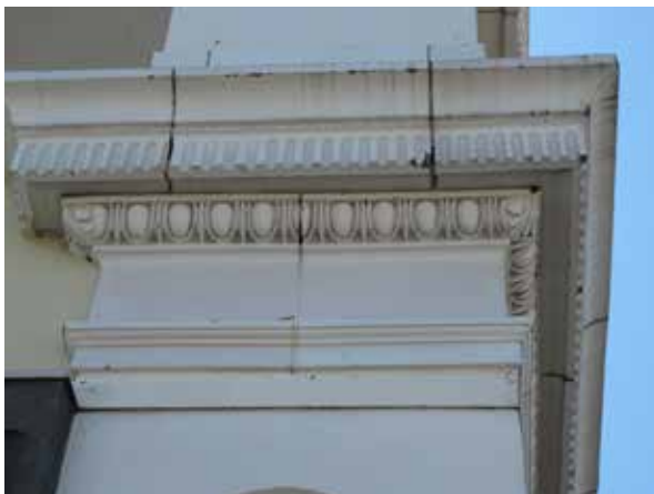
Above and Below: Glazed terra cotta storefront level cornice. Plain frieze with egg and dart and flute mouldings. Staining, chips to finish, mortar loss and discoloured mortar typical of storefront cornice.
