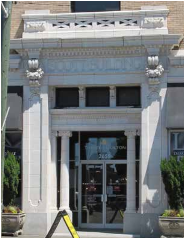
Above: Ornate portico of Douglas Street entry of terra cotta and granite.
