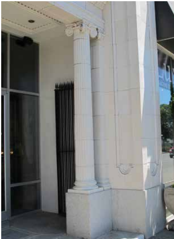
Above: Engaged square column with volute capital and Ionic column with volute capital on grey granite base present on both sides of Douglas Street entry. Metal security gates are a later intervention
