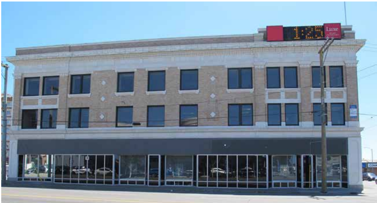
Above: Buff brick laid in running bond with light coloured mortar. Brick is present on the second and third floors, and parapet of primary façades.
