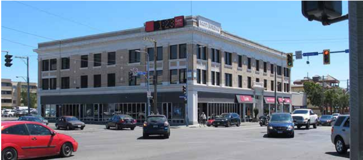
Three storey Scott Building with full-height storefront, brick and terra cotta exterior, and parapet.
