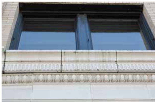
Above and Below: Glazed terra cotta storefront level cornice. Plain frieze with egg and dart and flute mouldings. Staining, chips to finish, mortar loss and discoloured mortar typical of storefront cornice.
