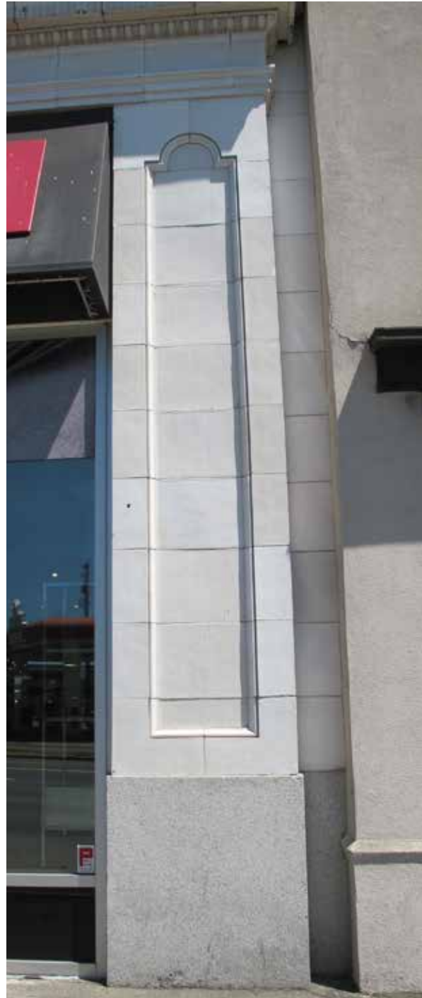
Above: Example of storefront level column clad in glazed terra cotta with sunk panel. Typical materials and design of intact storefront level columns.
