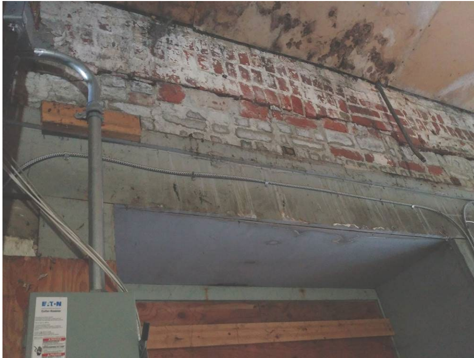
Segmental arch above altered front opening
