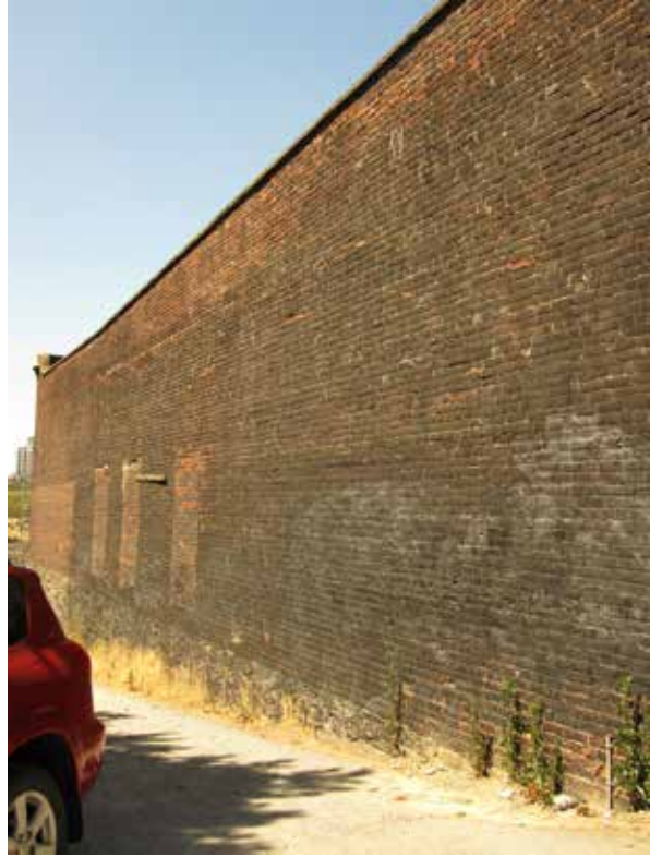
Current south Elevation of the Caire & Grancini Warehouse
