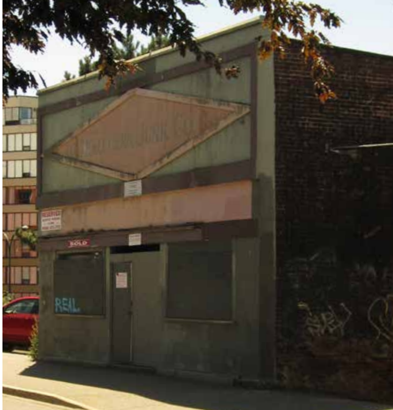
Current front elevation of the Caire & Grancini Warehouse
