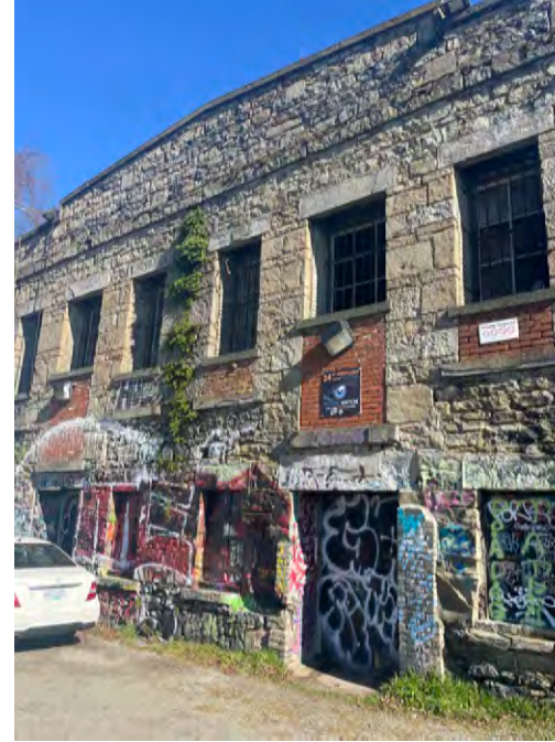
FRASER WAREHOUSE EAST FACADE
