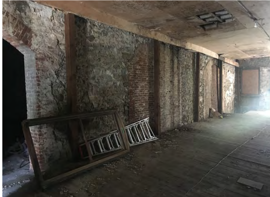
EXISTING INTERIOR CONDITION
