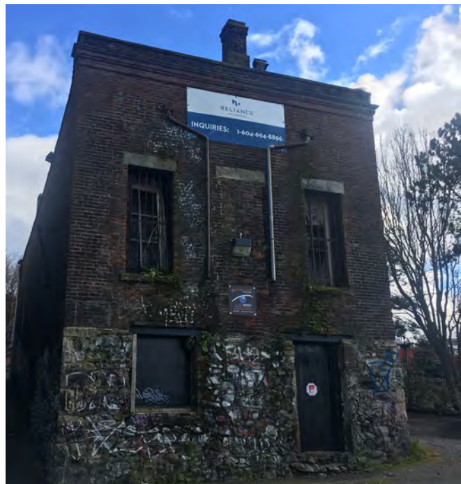
EXISTING CAIRE & GRANCINI WEST FACADE
