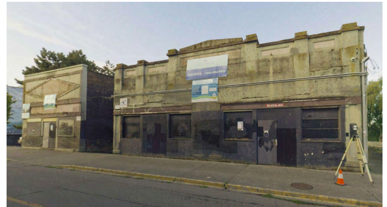
EXISTING EAST FACADES
