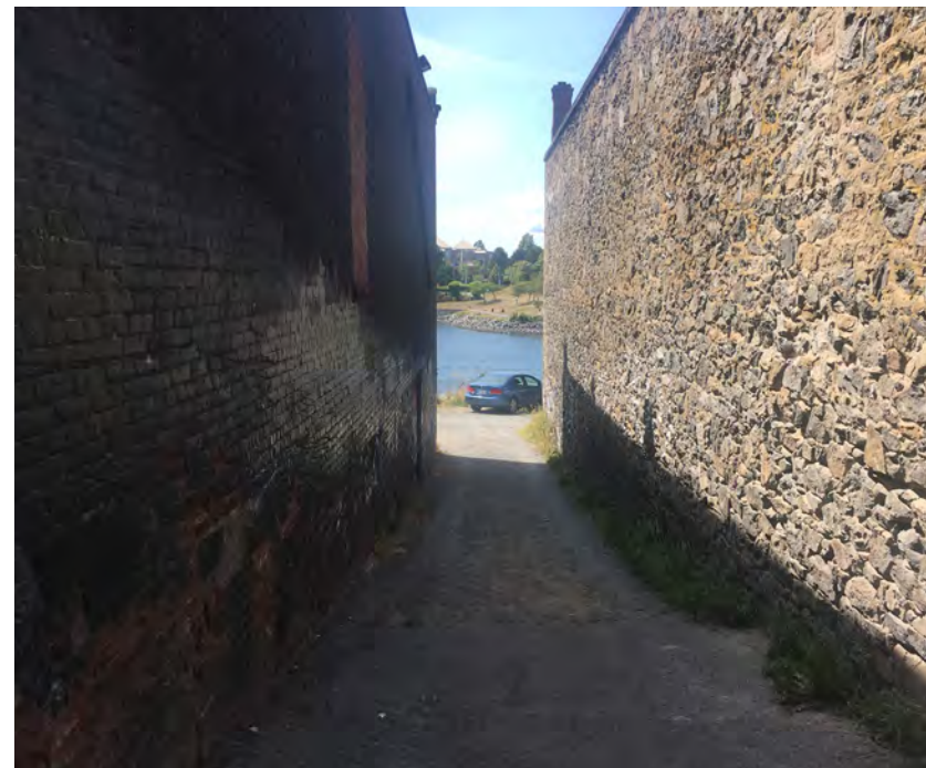
EXISTING ALLEYWAY BETWEEN BUILDINGS
