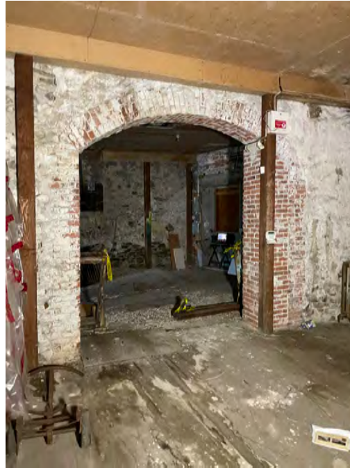
EXISTING INTERIOR CONDITION
