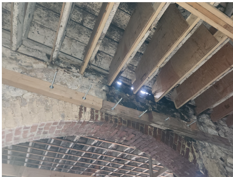
Figure 7 – Interior Roof Support Condition at Interior Bearing Wall
