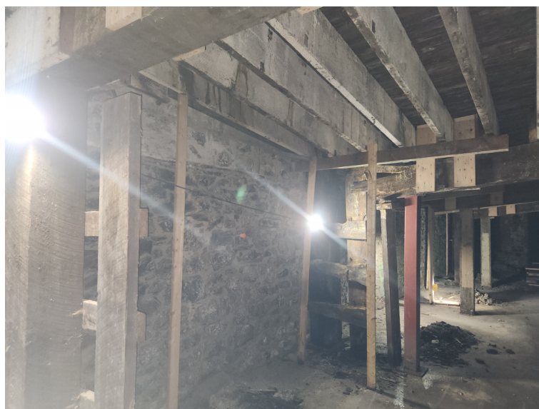
Figure 13 – Temporary Floor Framing Supports
