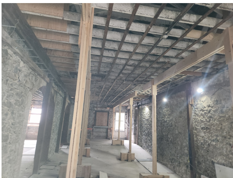
Figure 11 – Temporary Roof Framing Supports at North Wall
