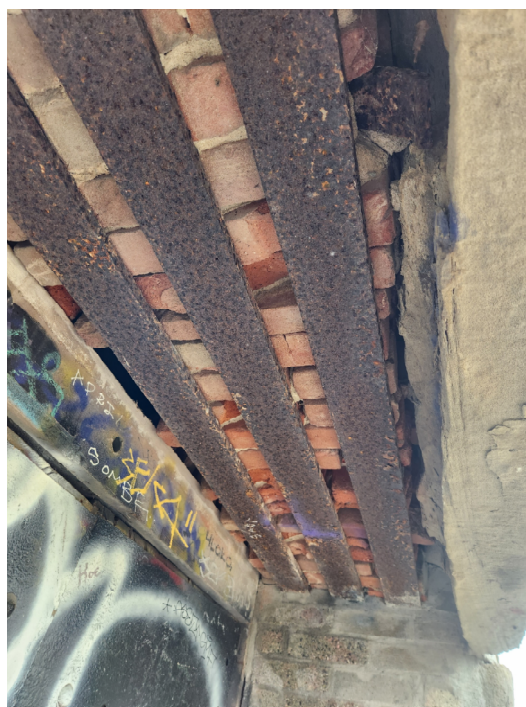
Figure 15 – Window Header Supports in West Wall
