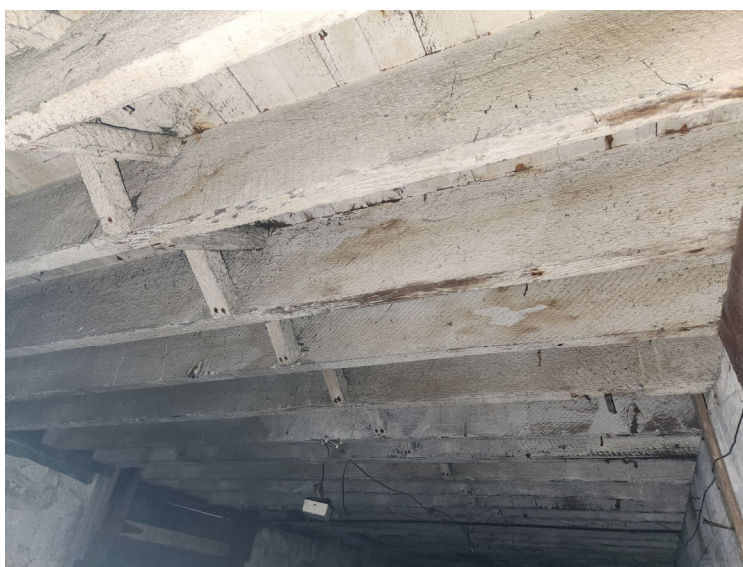
Figure 22 – Typical Floor Framing Soffit Layout
