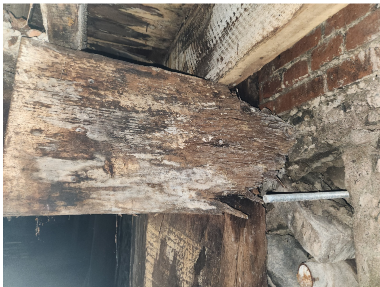
Figure 12 – Rotted Heavy Timber Support Beam
