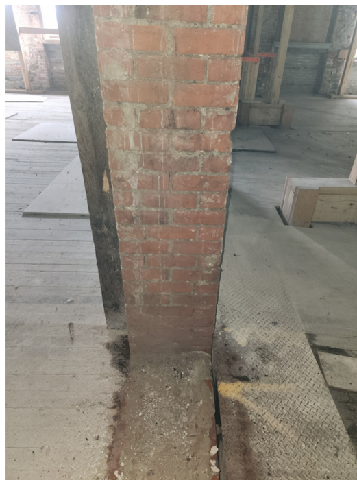
Figure 10 – Interior Wall Bricked Opening
