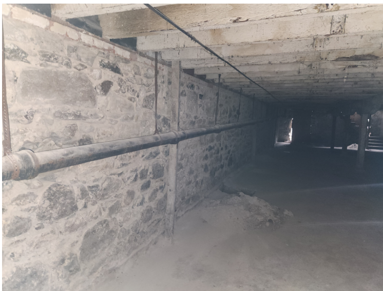
Figure 21 – South Stone Wall and Floor Framing Above at Basement
