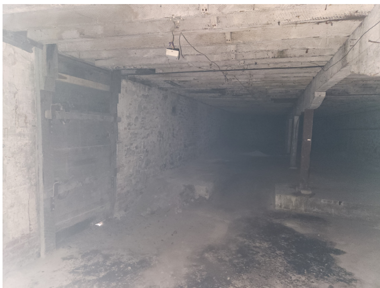
Figure 20 –North Stone Wall and Floor Framing Above at Basement
