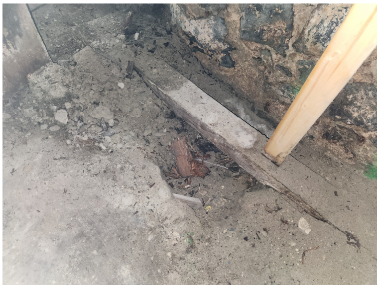
Figure 14 – Weathered Slab-on-Grade at Basement
