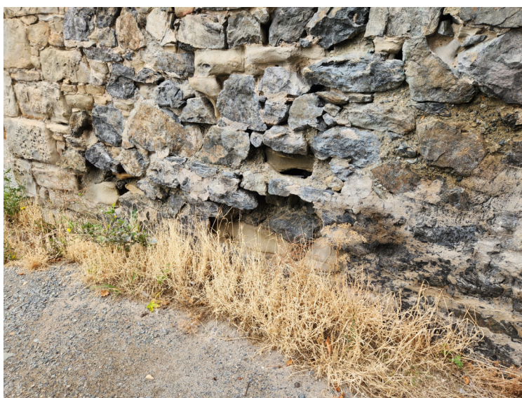
Figure 6 – Extremely Deteriorated Condition of Sandstone in Exterior Walls
