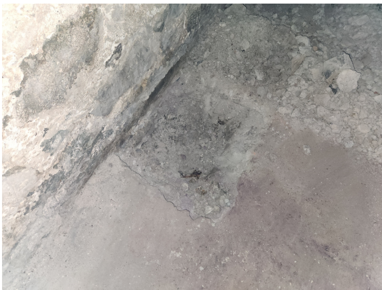
Figure 23 – Weathered Slab-on-Grade at Basement
