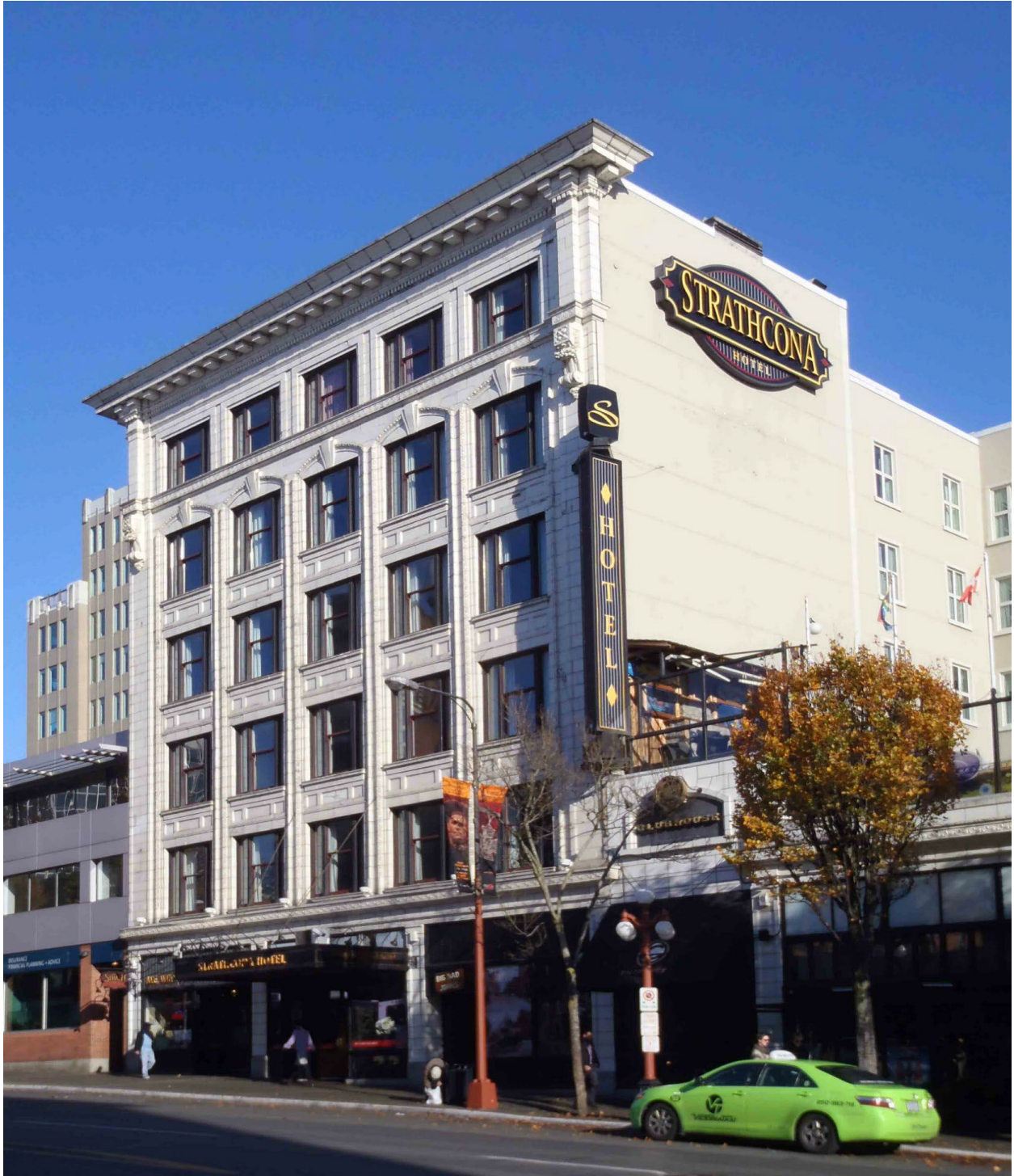
Strathcona Hotel, 919 Douglas Street . Designed by Henry S. Griffith in 1911.
