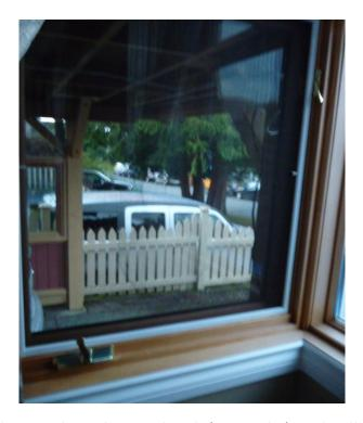
The windows have a hook (top right) and roll out handle (lower left) which lock the window. The window has a screen, (white frame). The window can only be opened from inside by releasing the hook and rolling the window open with the handle.
