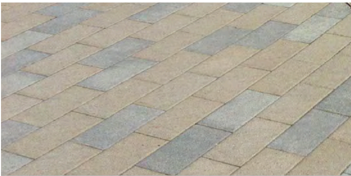
CONCRETE UNIT PAVING
