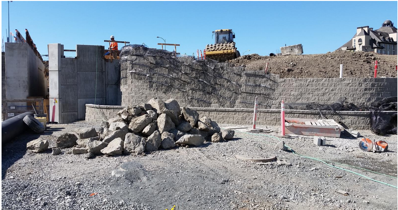
Wall 11 can be seen curving to the right during construction with stabilizing geogrid ready for installation. Seen on the left: Wall 4 (west abutment) precast panels coming to final elevation.
