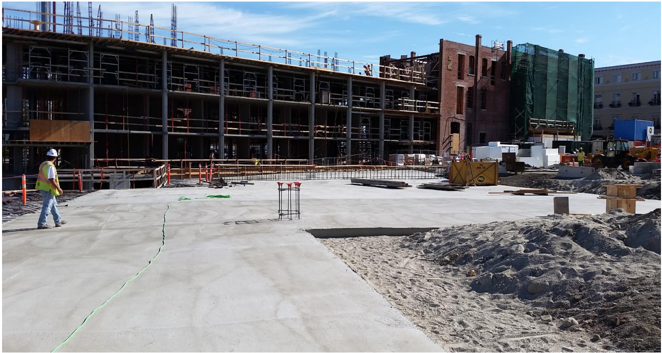
The structural concrete slab poured over the EPS foam blocks; Janion in the background.
