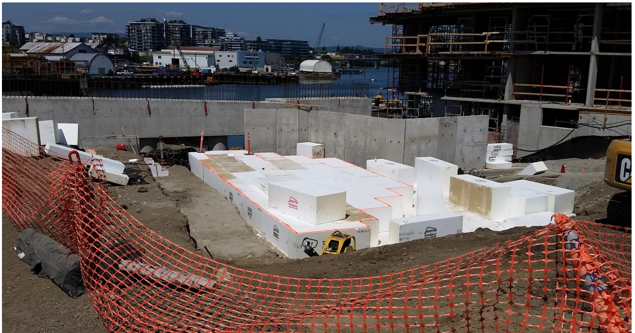
Foam EPS blocks can be seen during installation with the Janion to the right and Point Hope Shipyard in the distance.
