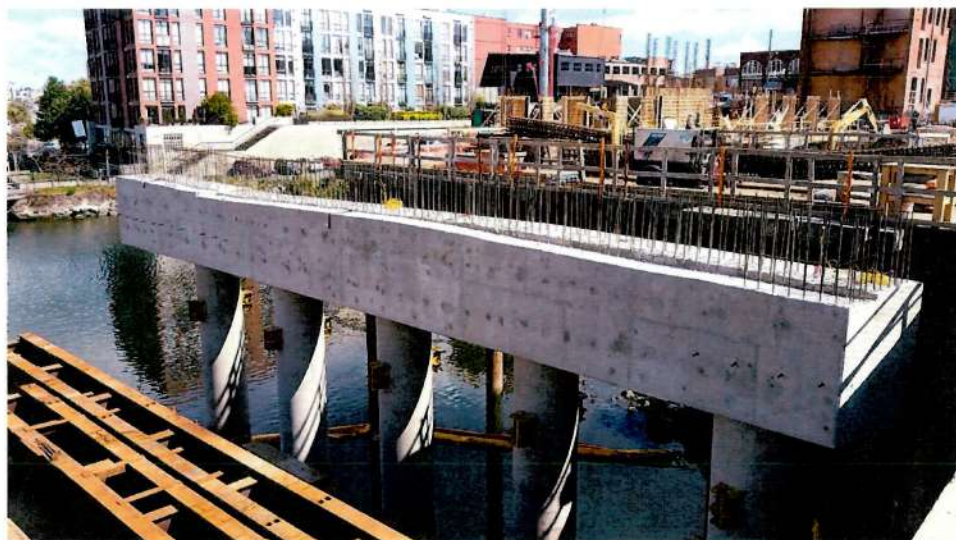
Intermediate pier on the east side (between shore and bascule)
