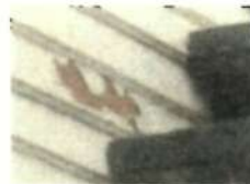
PAINTED EX 6" BEADED SHIPLAP SIDING.
