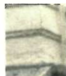
PAINTED EX 6" BEADED SHIPLAP SIDING.
