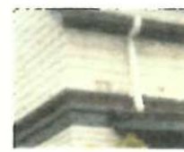
PAINTED COMMON COURSED SAWN CEDAR SHINGLES WITH TAPER. PAINTED EX 8" BEADED SHIPLAP SIDING.
