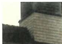
PAINTED COMMON COURSED SAWN CEDAR SHINGLES WITH TAPER.
