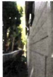
EX 8" SHIPLAP SIDING, PLYWOOD BOARD
