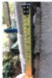
PAINTED EX 6" BEADED SHIPLAP SIDING.
