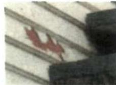
PAINTED EX 6" BEADED SHIPLAP SIDING.
