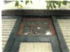
PAINTED COMMON COURSED SAWN CEDAR SHINGLES WITH TAPER, PAINTED EX 6" BEADED SHIPLAP SIDING.
