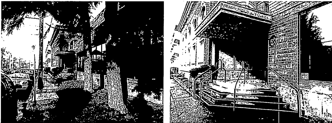
Location of proposed one storey lobby addition. Reduced setback would not feel out of character along the north side of North Park. Existing stairs are steep and not accessible. Area to be enclosed and ramp access created from new lobby.
