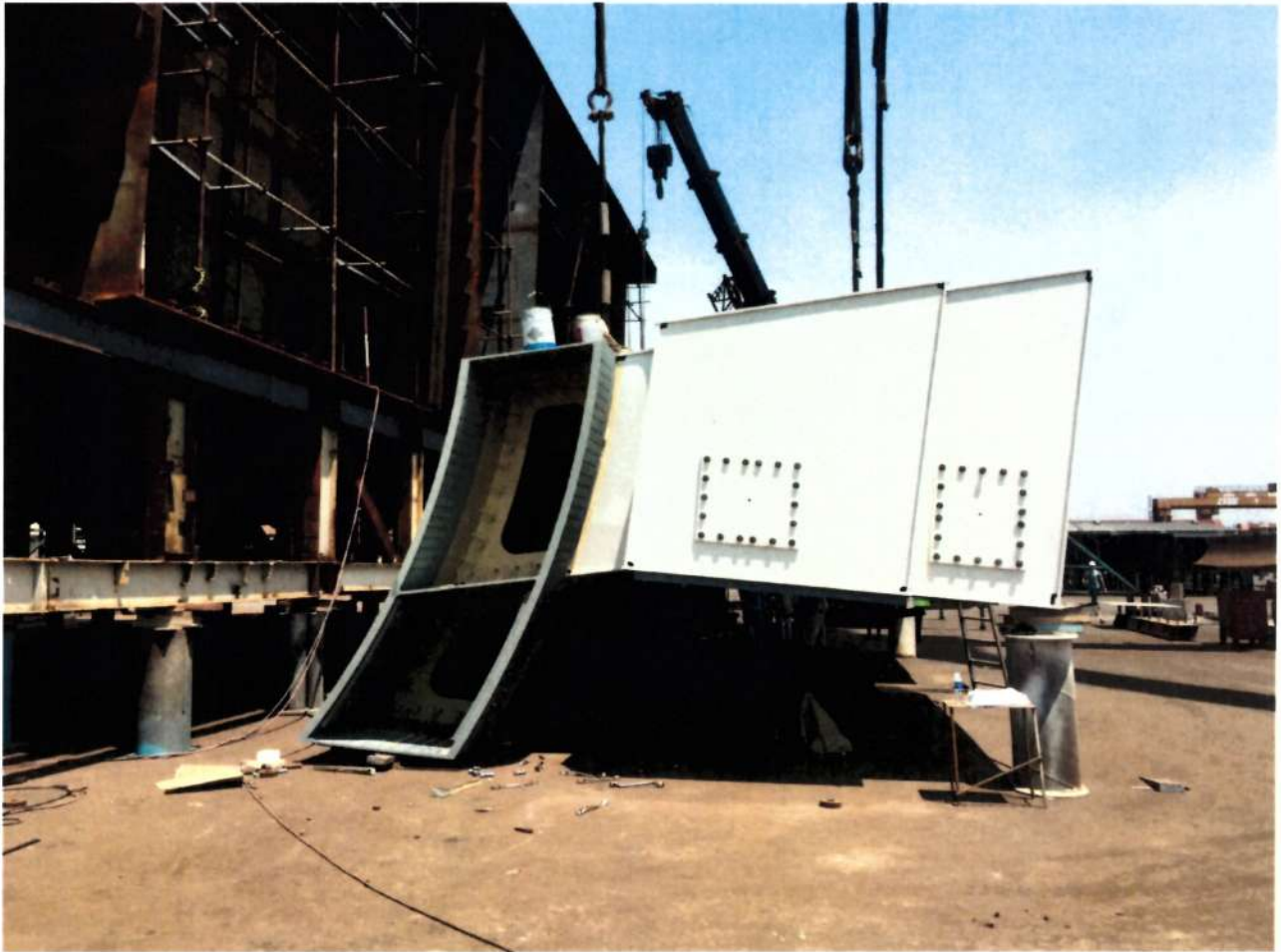
Figure 2 – Lower Counter Weight prior to loading
