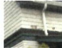
PAINTED COMMON COURSED SAWN CEDAR SHINGLES WITH TAPER, PAINTED EX 6" BEADED SHIPLAP SIDING.
