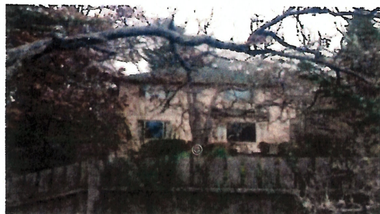
Elevation 615 Foul Bay
