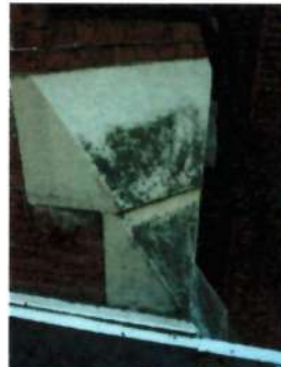
10. Detail of water drainage system, north elevation. These have been moved with the restoration, taking into the use of the water as water drainage system
