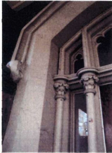
Photo above: Sandstone door surround with partially-covered hood mould. Note carved entrance door assembly.
