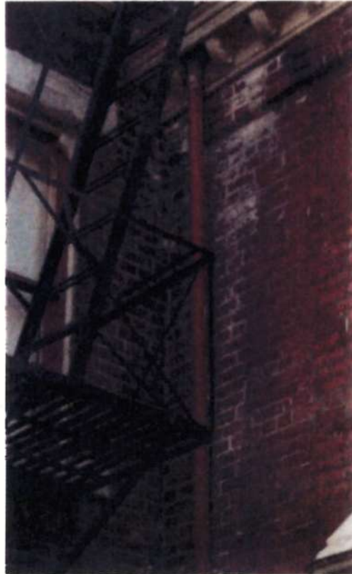
Example of efflorescence on brick from many wetting-and-drying cycles due to a faulty downspout. North elevation
