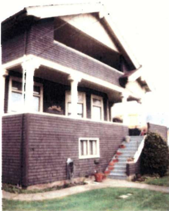
Clockwise: (top) South elevation with open verandah and sleeping porch; sleeping porch; verandah with wood columns and tongue & groove soffits.
