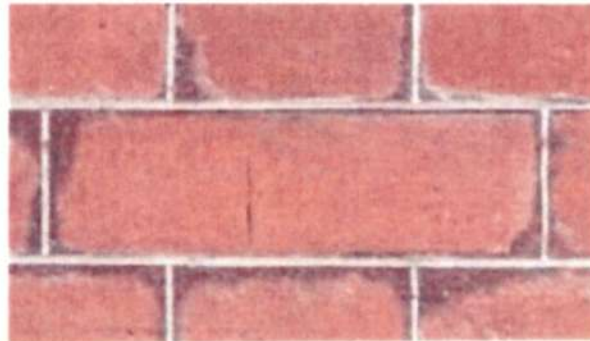
Example of typical completed tuck-pointing on another building.
