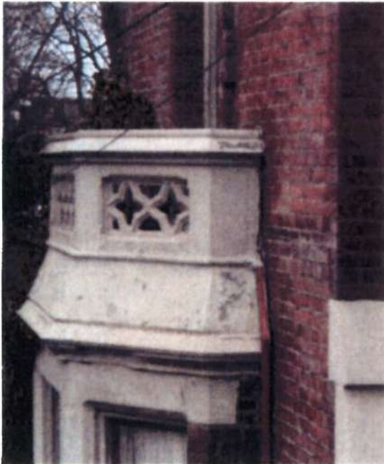
Sheet metal flashing on balcony. Substrate unknown. West elevation
