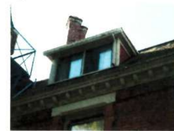
8. The dormer would be restored and related with the roof. The roof would be replaced with the original gabled roof
