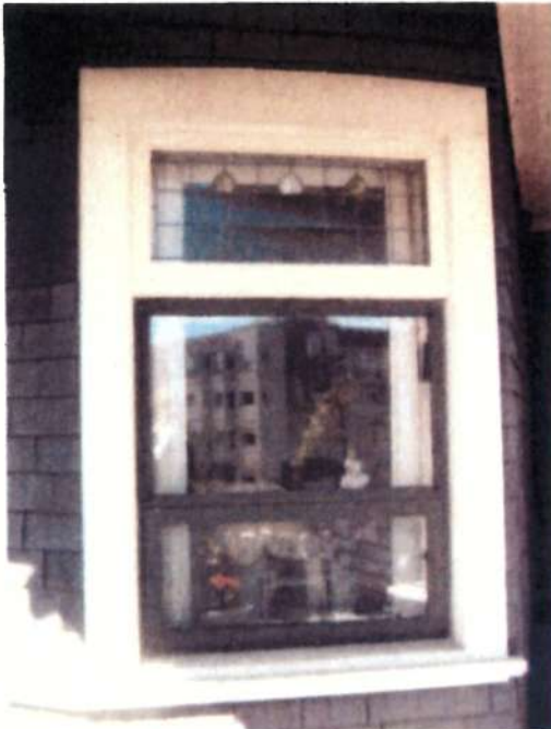
The original window trim, sill and sash of the former double-hung window and the hinged transom with stained glass are retained. A historically inappropriate aluminum unit was installed.
