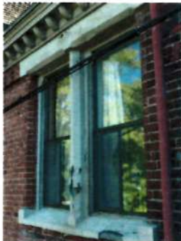
24. window ribs and frames are in poor condition in some areas. Severe water damage and missing ribs are also visible. Severe water damage is also visible.
