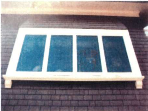
Bay window with a quadruple casement assembly and stained glass, east elevation.
