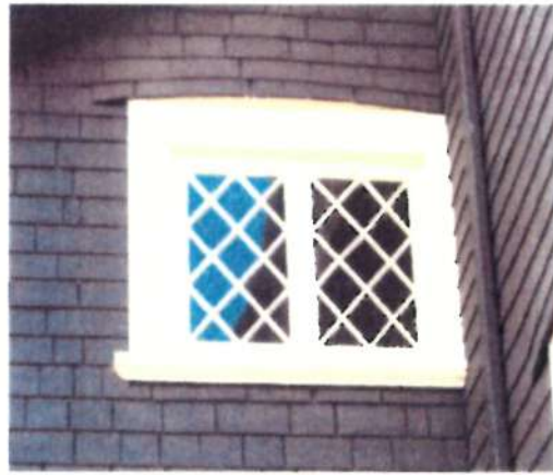
Fixed lattice window with typical window hood on the north elevation.
