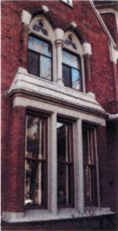
Photo above: Condition of sandstone. Minor deterioration under paint layers causes cracking of paint and therefore moisture ingress
