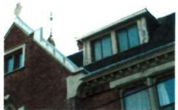
20. detail of gable and corner. The battens are in fair condition.
