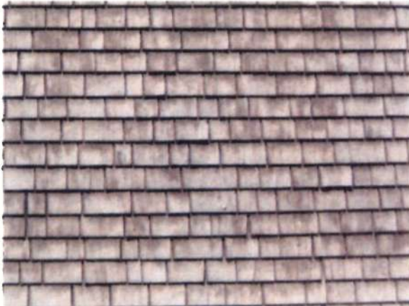
Typical square butt wood shingles.
