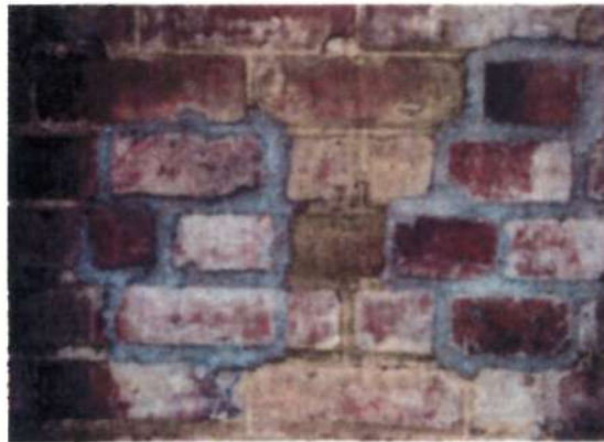
Example of inappropriate repointing using cement-based mortar, exaggerating the joints
