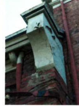
28. water damage to masonry. The gable battens above would be replaced as part of the restoration.
