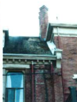
26. west wall, detail showing water damage. Chimney would be rebuilt.
