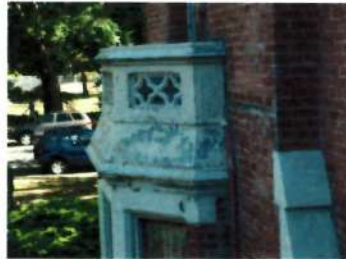
19. detail of bay window. Missing metal reveals severely deteriorated. The casting on the window sill is missing.
