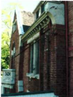
18. detail of west wall. Separation of the masonry ribs and window frames is evident. As is water damage below the gable. The original building stepped back at this point.
