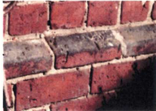
Photo above: Cant brick at plinth level.
