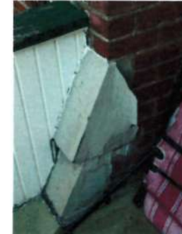
23. detail of masonry. Water absorption. Water seeps in the absorption causing a loss of the masonry in the corner.
