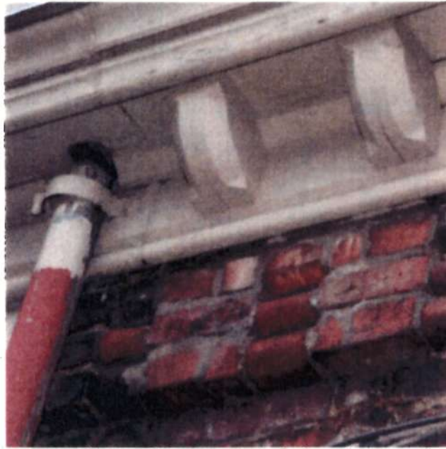
Downspout disconnected from eavetrough, allowing moisture saturation. Brick cornice previously repaired but downspout not repaired. Note wood cornice with brackets split at dowels from moisture
