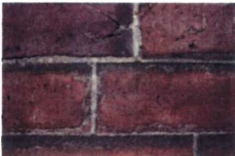
Photo above: Detail of remaining tuck-pointing in sheltered area of Angela College.
