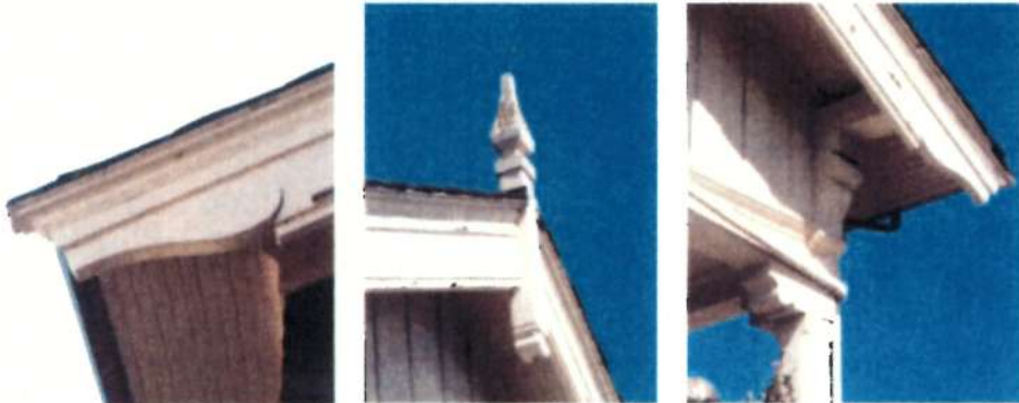
Woodwork details: (top): Decorative woodwork at south gable; (from left to right): milled bargeboard ends; finials; brackets and capitals.
