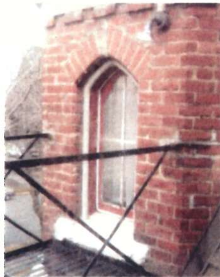
Photo above: Detail of remaining tuck-pointing in sheltered area of Angela College.
