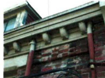
27. detail of water damage. West side. Two sets of iron water fixtures show an attempt to make the problem in this area.
