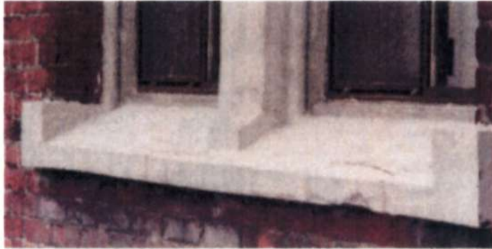
Photo above: Condition of sandstone. Minor deterioration under paint layers causes cracking of paint and therefore moisture ingress
