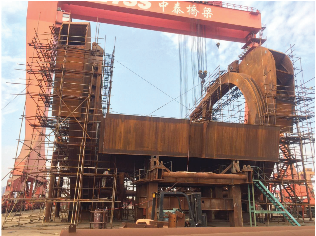
Figure 2 - Vertical Fit Up – Back View Showing Lower Counter Weight as of 16 March 2017
