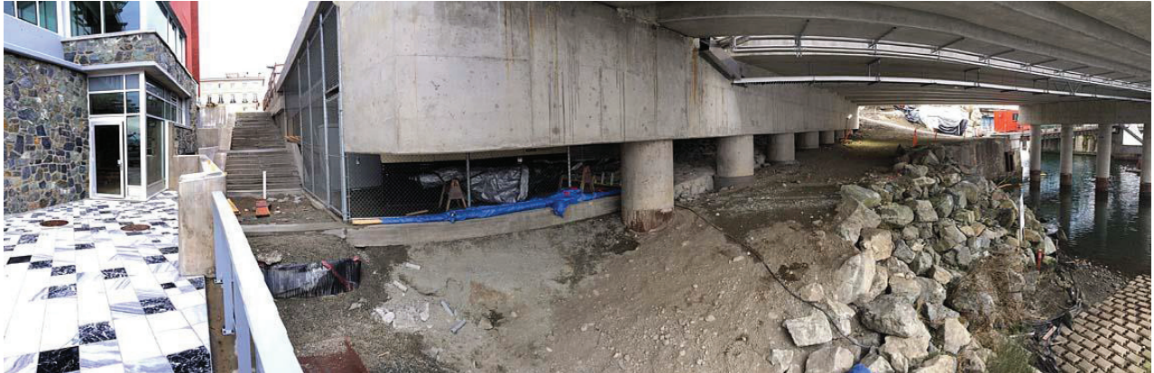
Image: stairs leading from Janion plaza between Janion building and new JSB
