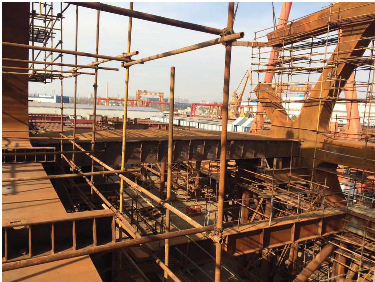
Figure 3 – Side View of Vertical Fit Up as of 16 March 2017
