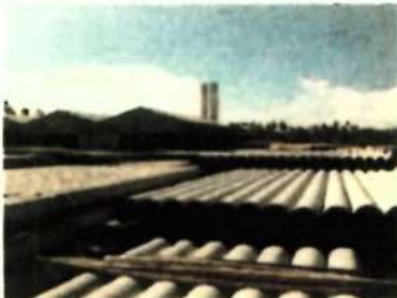
5: Concrete Plings painted black to be used for the Seawall
