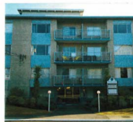
3 PHOTO 2 - OVERALL BUILDING VIEW A-007
