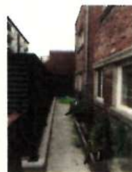
Courtyard Building South Side
