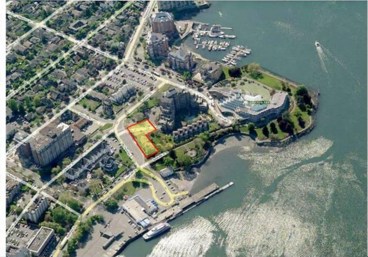
AERIAL VIEW FROM NORTH
