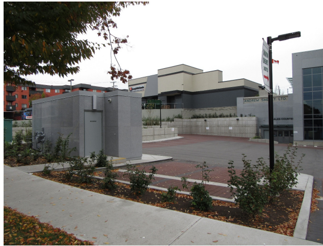
740 Hillside – DVP # 00157 – Rear Parking Area
