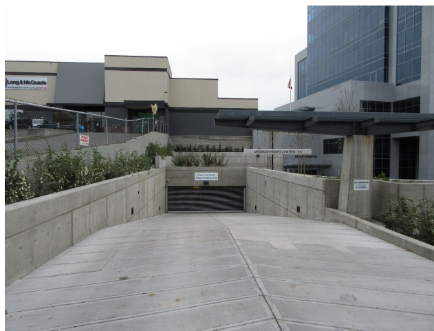
740 Hillside – DVP # 00157 – Ramp to Underground Parking Level
