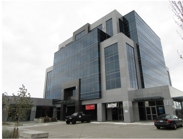
740 Hillside – DVP # 00157 – Front Parking Area (Hillside Ave.)
