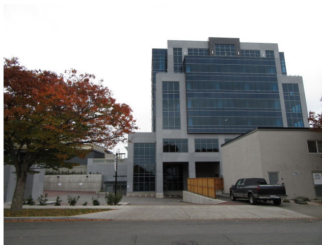
740 Hillside – DVP # 00157 – Entrance to Rear Parking Area
