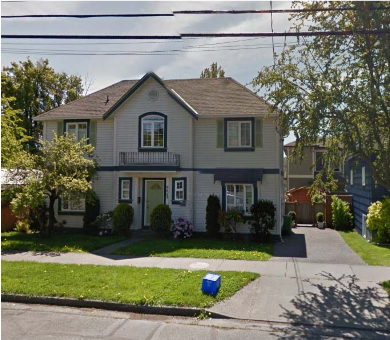
Properties to the West – Single Family Dwelling
