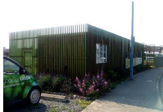
West Elevation & Access Gate
