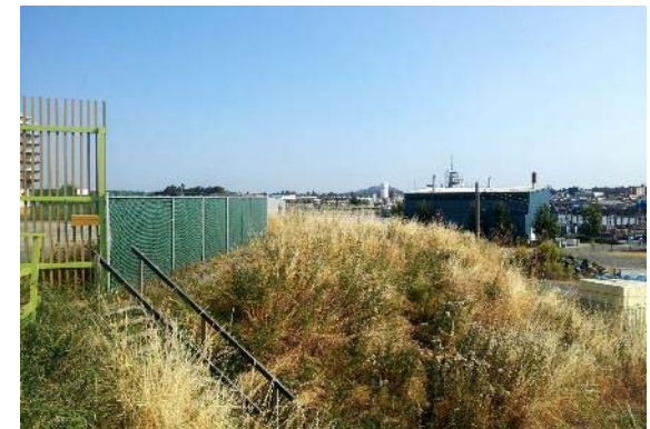
Back Stair to Harbour Rd
