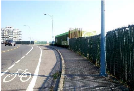
Tyee Rd Street Frontage
