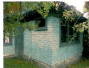
DET. TRANSCOM WINDOW WINDOW TO BE RESTORED TO INCLUDE LEADED GLASS TYPICAL OF ORIGINAL CHARACTER
