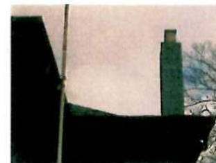
BRICK CHIMNEY (NOT ORIGINAL) CHIMNEY LEAVING BRICK CHIMNEY TO BE REMOVED AND RECONSTRUCTED IN STONE TYPICAL OF ORIGINAL CHARACTER
