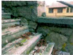
WEST WALL OF MAIN ENTRANCE STAIR SIGNIFICANT CRACKING IN STONE MASONRY STONE MASONRY TO BE RECONSTRUCTED & NEW SUPPORT CONSTRUCTED FROM BENEATH PAINT TO BE REMOVED FROM MAIN PORCH & FRONT ENTRY CONCRETE CAPS OVER STONE CAPS TO REMAIN UNPAINTED
