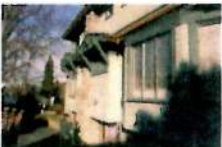
CEDAR SHINGLE CLADDING AND ROUGH CAST STUCCO ABOVE
