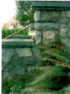
WEST WALL OF MAIN ENTRANCE STAIR SIGNIFICANT CRACKING IN STONE MASONRY STONE MASONRY TO BE RECONSTRUCTED & NEW SUPPORT CONSTRUCTED FROM BENEATH PAINT TO BE REMOVED FROM MAIN PORCH & FRONT ENTRY CONCRETE CAPS OVER STONE CAPS TO REMAIN UNPAINTED
