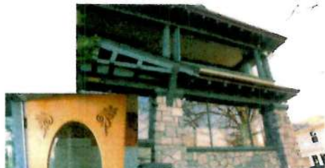
FRONT ELEVATION SHOWING GRANITE STONE FOUNDATIONS & PILLARS
