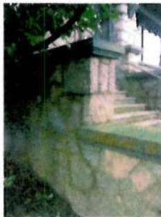
EAST WALL OF MAIN ENTRANCE STAIR CRACKING IN STONE MASONRY STONE MASONRY TO BE RECONSTRUCTED & NEW SUPPORT CONSTRUCTED FROM BENEATH
