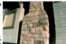
STONE GRANITE STONE CHIMNEY & CEDAR SHINGLE CLADDING
