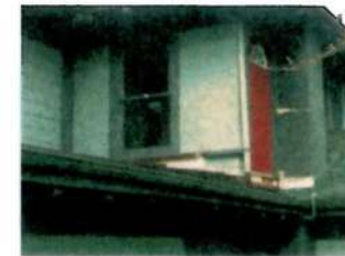
HISTORIC SITTING ROOM EXISTING DOUBLE HUNG WINDOW TO BE REPAIRED AND RESTORED WITH WINDOW TYPICAL OF ORIGINAL CHARACTER WINDOW TO MATCH OPPOSITE SIDE
