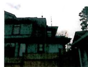
SOUTH WEST CORNER ROOFLINE LOWER ROOF TO BE RECONSTRUCTED TO CORRECT CHARACTER OF HISTORIC PORCH AREA ROOF OVERHANG AT SECOND FLOOR TO BE RESTORED TO MATCH PERIODIC DETAILING
