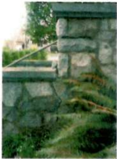
WEST WALL OF MAIN ENTRANCE STAIRS CONCRETE CRACKS IN STONE MASONRY STONE MASONRY TO BE RECONSTRUCTED & NEW SUPPORT CONSTRUCTED FROM PAINTED PAINT TO BE REMOVED FROM MAIN PORCH & FRONT ENTRY CONCRETE CAPS OVER STONE CAPS TO REMAIN UNPAINTED
