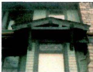
ARTS & CRAFTS STYLE GABLE WORK TO INCLUDE STRENGTH & NEW PAINT NEW FINISHES TO BE INSTALLED OVER TOP OF BEAMS ENDS, ALL TYPICAL THROUGHOUT CONSIDER CHIMNEY COLOUR BEHIND GABLE BEFORE FINAL PAINTING
