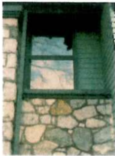
MAIN PORCH OPEN FRONT PORCH TO BE RESTORED GLAZING TO BE REPAIRED
