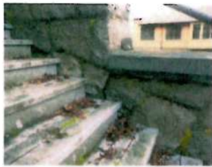
WEST WALL OF MAIN ENTRANCE STAIRS CONCRETE CRACKS IN STONE MASONRY STONE MASONRY TO BE RECONSTRUCTED & NEW SUPPORT CONSTRUCTED FROM PAINTED PAINT TO BE REMOVED FROM MAIN PORCH & FRONT ENTRY CONCRETE CAPS OVER STONE CAPS TO REMAIN UNPAINTED
