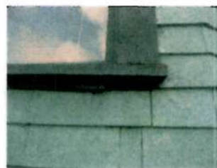
BAY WINDOW SILL CONDITION WINDOW SILL & CASINGS TO BE MAINTAINED, TYPICAL THROUGHOUT WORK TO INCLUDE STRENGTH AND NEW PAINT
