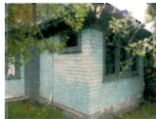
EAST ELEVATION HISTORIC WINDOWS TO BE RESTORED TO INCLUDE LEADED GLASS TYPICAL OF ORIGINAL CHARACTER
