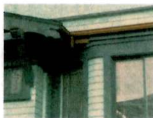
BAY ROOF OVER ROOF OVER BAY TO BE RECONSTRUCTED FOR APPROPRIATE OVERHANGS PREVENTION AND RE INTO GABLE ROOF TO MATCH TYPICAL DETAILING
