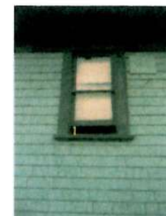
SOUTH WEST CORNER WINDOW WINDOW TO BE RECONSTRUCTED GLASS TO BE REPLACED WITH ORIGINAL TO SUIT NEW WASHROOM PANEL BEHIND TO BE REPAIRED AND WINDINGS TO BE RESTORED
