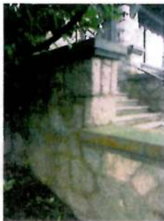
WEST WALL OF MAIN ENTRANCE STAIRS CRACKS IN STONE MASONRY STONE MASONRY TO BE RECONSTRUCTED & NEW SUPPORT CONSTRUCTED FROM BENEATH
