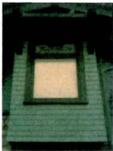
LEADED GLASS WINDOW WINDOW IN RELATIVELY GOOD CONDITION REPAIRS TO BE PERFORMED AS REQUIRED
