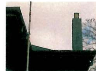
BRICK CHIMNEY (NOT ORIGINAL) CHIMNEY TO BE REMOVED AND RECONSTRUCTED IN STONE TYPICAL OF ORIGINAL CHARACTER
