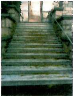
MAIN ENTRANCE STAIRS WOODEN STEPS TO BE RECONSTRUCTED NEW STEPS TO BE CONSTRUCTED FROM PAINTED TIMBER MATERIAL WITH SINGLE GAP, AND INTEGRAL BULLDOSE RAMPING TO BE FROM BELOW BY BRACKETS RESTORATION OF NEW FRONT STEPS TO BE MORE IN KEEPING WITH ORIGINAL DETAILS
