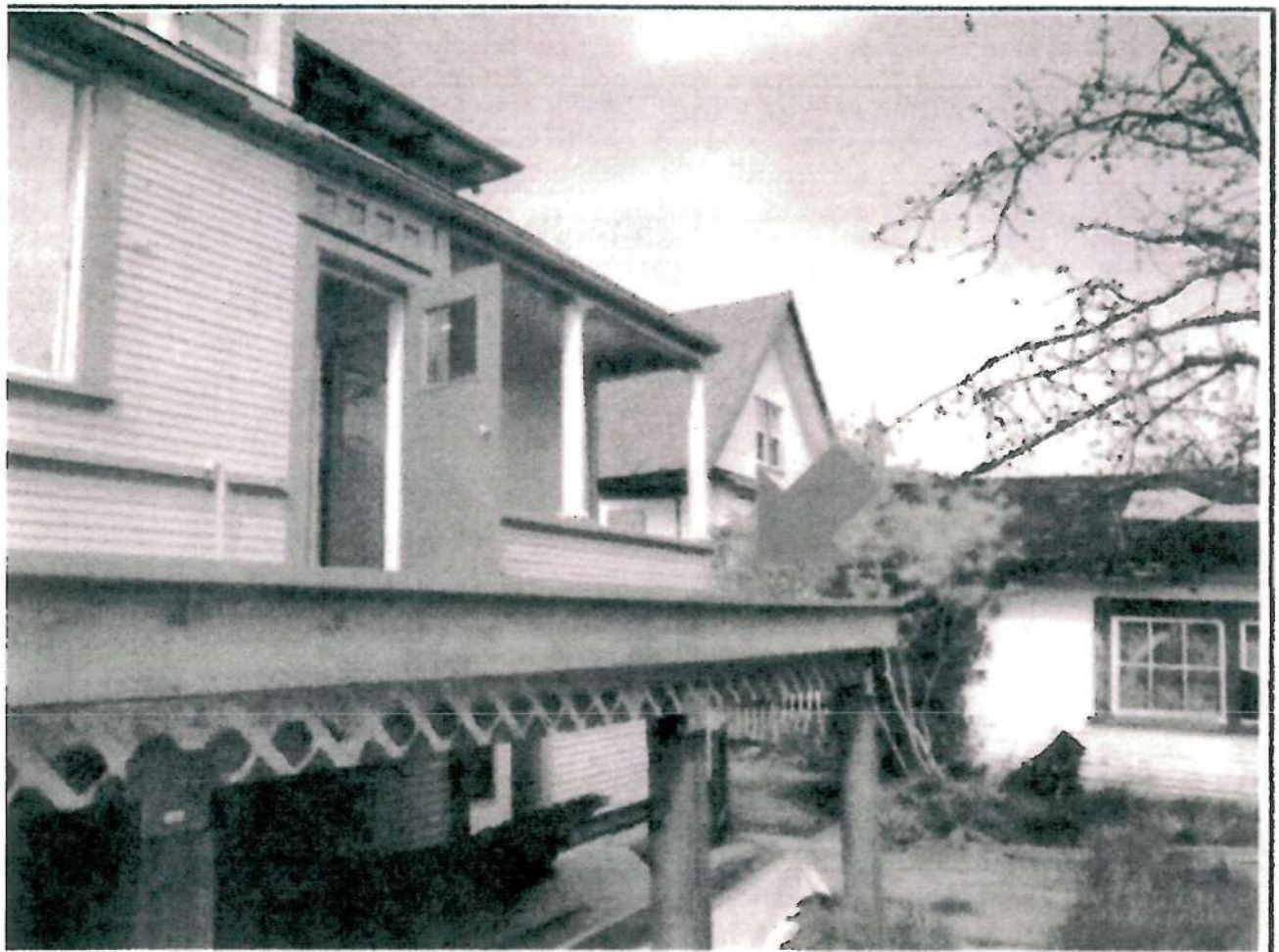
Photo 3: Rear deck of 135 Medana in 2012. The red arrow denotes lack of guardrails and stairs
