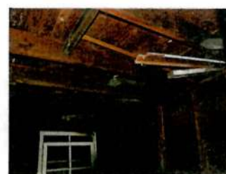
INTERIOR VIEWS, ROOF
