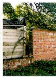
BRICK WALL, AT WEST ELEVATION
