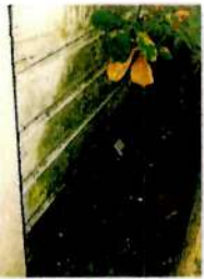
DETAIL OF NORTH WALL
