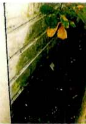
DETAIL OF NORTH WALL
