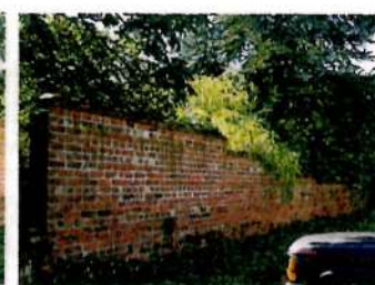
BRICK WALL TO WEST OF BUILDING
