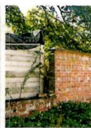
BRICK WALL AT WEST ELEVATION
