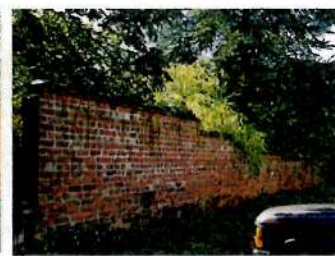
BRICK WALL TO WEST OF BUILDING
