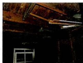
INTERIOR VIEWS, ROOF
