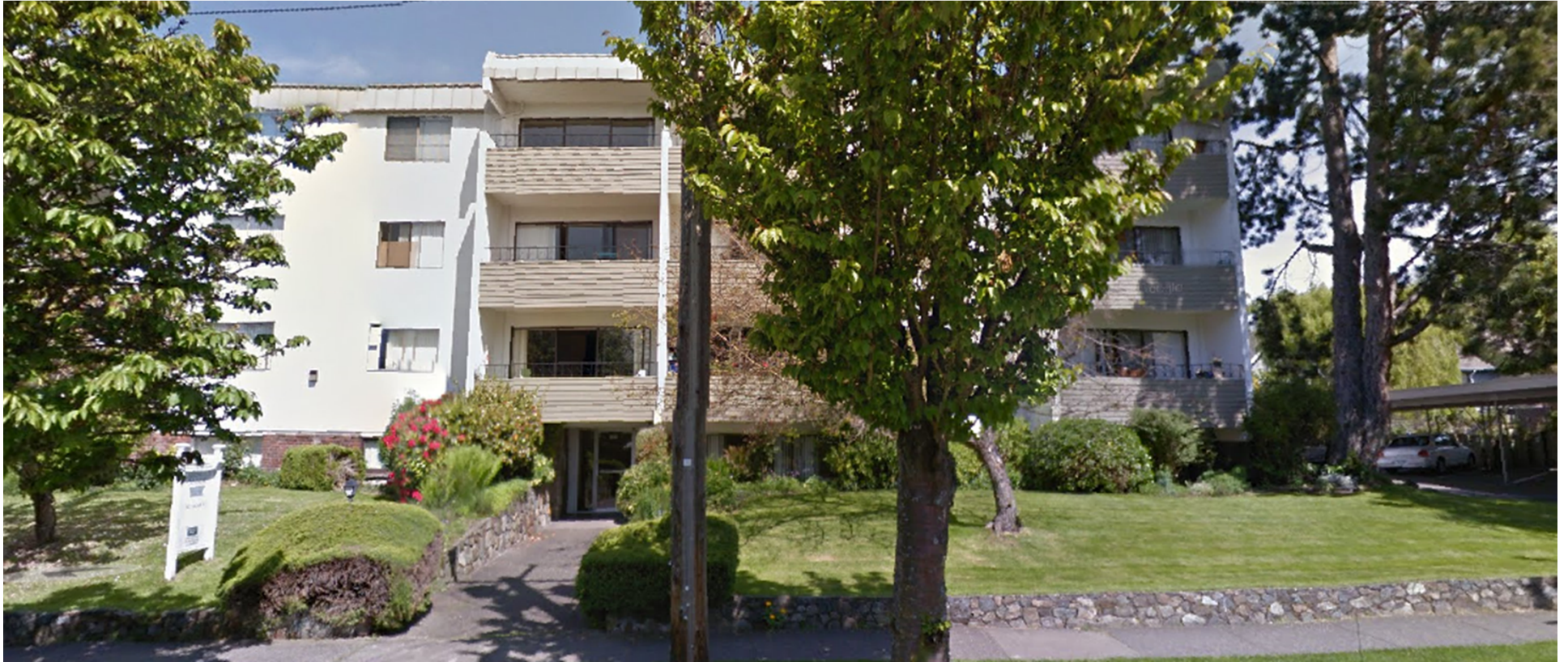
Property to the West – Four-Storey Apartment Building
