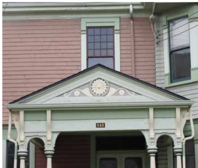
Wood detailing in front-gabled verandah roof.
