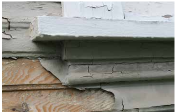
Condition of exterior painted wood surfaces.
