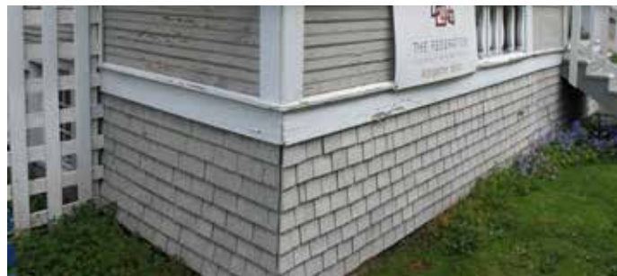
Shingle siding on foundation.
