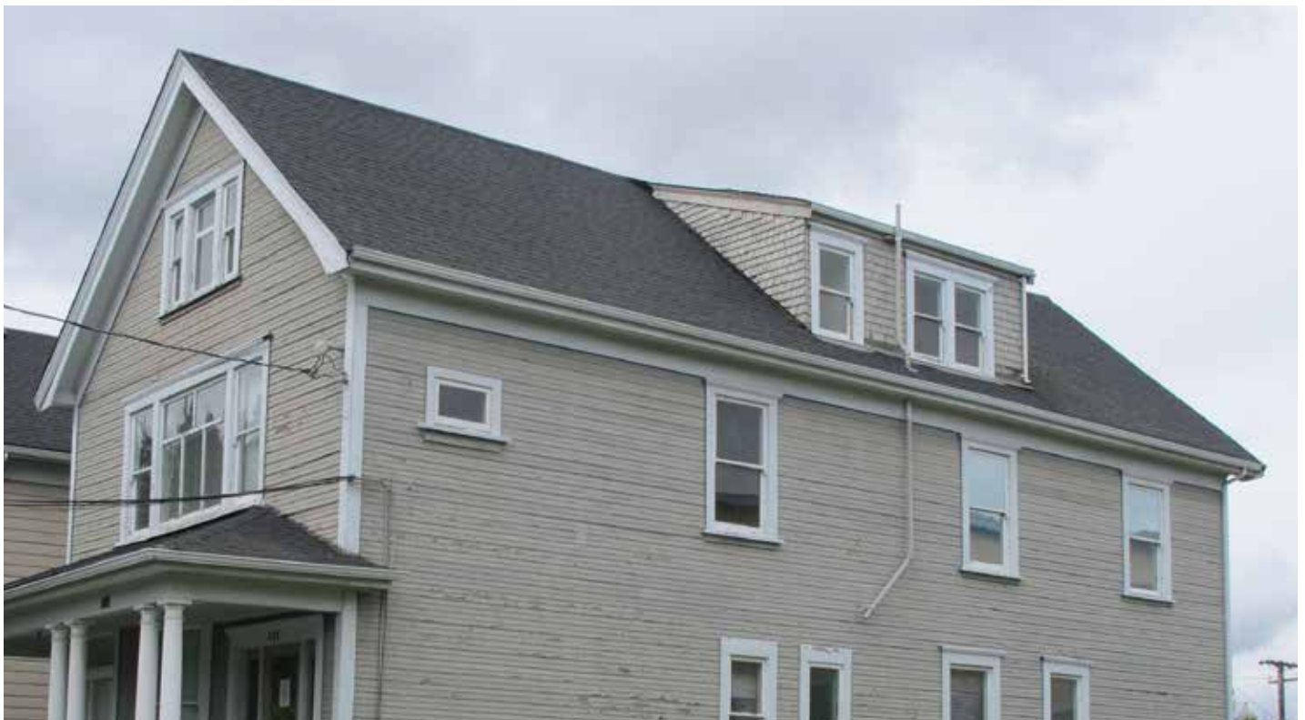
Roof configuration with shed dormer.
