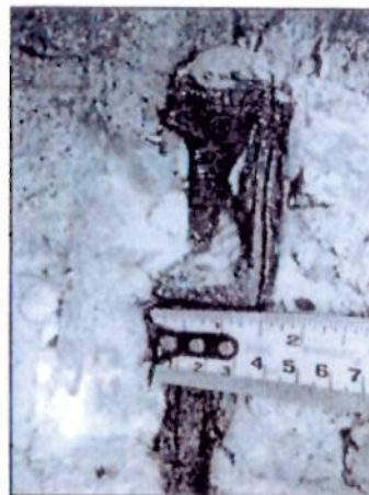
Photo 3- Corroded Outrigger
