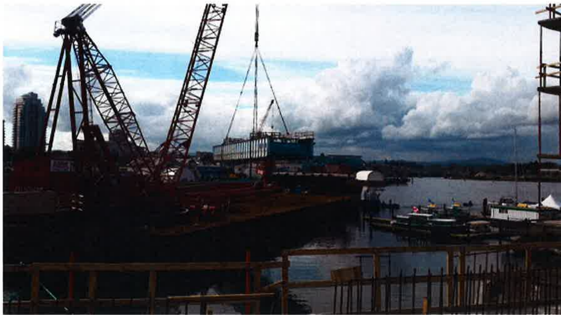
Arctic Tuk lowering the last rail span on the deck of its barge.
