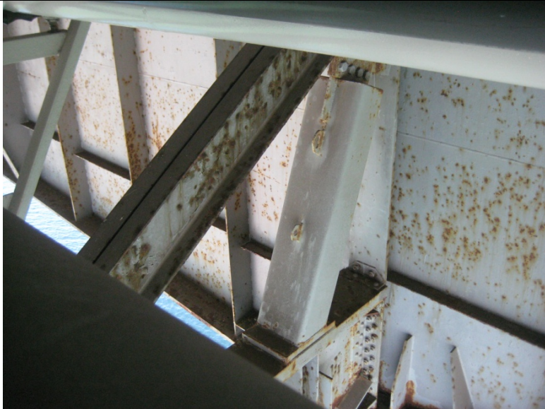
Photo 5 – Interior view of the North Girder near Pier #1. Surface corrosion and pitting is visible on steel elements.
