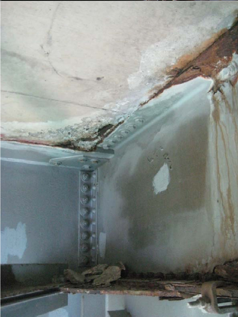
Photo 6 – Concrete spalling observed at the connection point of the cross beam and stringer
