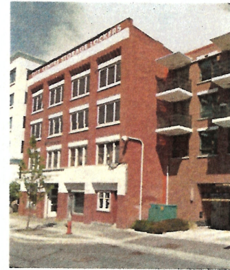
3 Exterior Photo - East Face of Exterior
