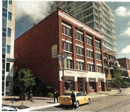
1 Exterior Photo - West Face of Exterior
