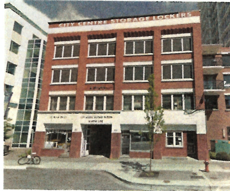
2 Exterior Photo - South Face of Exterior
