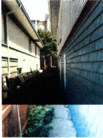
VIEW FROM WEST SIDE OF THE PROPERTY LOOKING EAST
