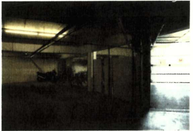
AUG. 01/17 6:30PM LEVEL B-2 (EXIT GATE)
