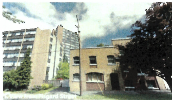
3. View from Plegard Street
