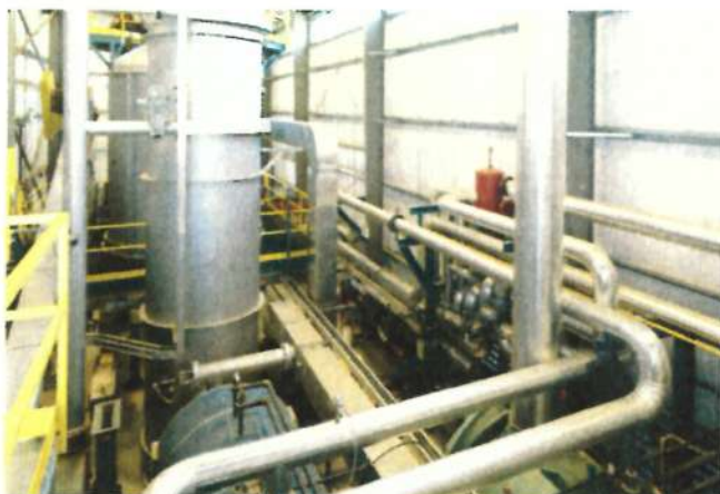
Dockside Green's biomass gasification system showing fuel feed (far left) to gasifier (background); oxidizer and hot water heater are in foreground.
