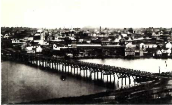
The Site: 1900 James Bay bridge replaced with causeway. The water flats were filled and 3,353 piles driven 125 feet to bedrock.
