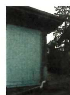
SOUTH WEST CORNER HISTORIC PORCH ENTRANCE PORCH (ADJACENT TO THE SOUTH) STRUCTURE TO BE MAINTAINED AND STRENGTHENING TO BE PROVIDED VERTICAL SILLING TO BE MAINTAINED AND SHINGLE CLADDING TO BE RESTORED
