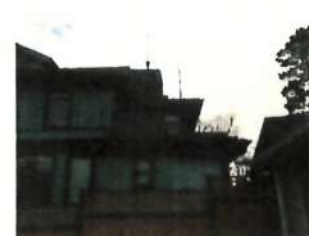
ROOF LINING LOWER ROOF TO BE RECONSTRUCTED TO CORRECT DRAINAGE OF ROOFING, PATCH AREA
