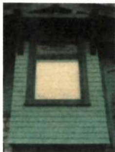
LEADED GLASS WINDOW WINDOW IS RELATIVELY GOOD CONDITION RELEADING TO BE PERFORMED AS REQUIRED
