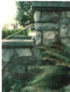
WEST WALL OF MAIN ENTRANCE STAIR STAIR PLANT WALLING IN STONE MASONRY STONE MASONRY TO BE RECONSTRUCTED & NEW SUPPORT CONSTRUCTED FROM BENEATH PAINT TO BE REMOVED FROM MAIN PORCH & FRONT ENTRY CONCRETE CAPS OVER STONE CAPS TO REMAIN UNPAINTED
