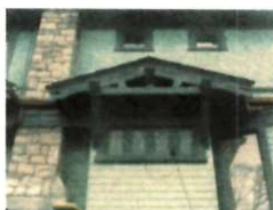
ARCH & CRAFT STYLE GABLE & LEADED GLASS WINDOW FLASHING TO GABLE AS PREVIOUSLY NOTED RELEASED TO BE PERFORMED AS REQUIRED THIRD PANE IN POOR CONDITION AND TO BE RESTORED
