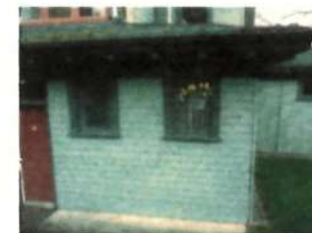
SOUTH EAST CORNER CONDITION EXTERIOR IN GOOD CONDITION, WALL CLADDING & ROOF TO BE MAINTAINED
