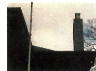
BRICK CHIMNEY NOT VISIBLE CHIMNEY LEANING BRICK CHIMNEY TO BE REMOVED AND RECONSTRUCTED IN STONE TYPICAL OF ORIGINAL CHARACTER
