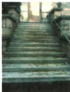
MAIN ENTRANCE STAIR WOODEN STEPS TO BE RECONSTRUCTED NEW STEPS TO BE CONSTRUCTED FROM PAVED 20mm MATERIAL WITH SINGLE GAP AND INTEGRAL BALUNDE, FASTENING TO BE FROM BELOW BY BRACKETS RESTORATION OF NEW FRONT STEPS TO BE MORE IN KEEPING WITH ORIGINAL DETAIL
