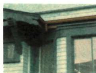
BAY ROOF OVER ROOF OVER BAY TO BE RECONSTRUCTED FOR APPROPRIATE OVERHANGING DETAILING AND TO MATCH GABLE ROOF TO MATCH TYPICAL DETAILING
