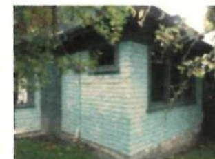
OLD TEA HOUSE WINDOW WINDOW TO BE RESTORED TO INCLUDE LEADED GLASS TYPICAL OF ORIGINAL CHARACTER
