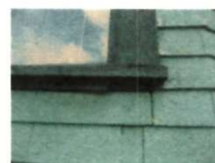
BAY WINDOW SILL CONDITION WINDOW SILL & CATCHES TO BE MAINTAINED, TYPICAL THROUGHOUT WORK TO INCLUDE SKIMMING AND NEW PAINT
