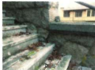
WEST WALL OF MAIN ENTRANCE STAIR STAIR PLANT WALLING IN STONE MASONRY STONE MASONRY TO BE RECONSTRUCTED & NEW SUPPORT CONSTRUCTED FROM BENEATH PAINT TO BE REMOVED FROM MAIN PORCH & FRONT ENTRY CONCRETE CAPS OVER STONE CAPS TO REMAIN UNPAINTED
