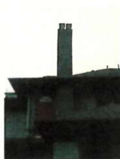
BRICK CHIMNEY AND WINDOW CHIMNEY TO BE REMOVED AND RECONSTRUCTED IN STONE TYPICAL OF ORIGINAL CHARACTER
