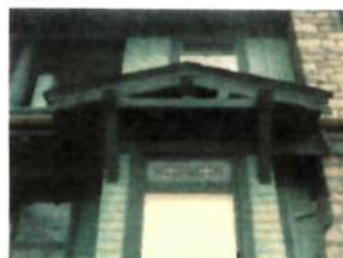
ARCH & CRAFT STYLE GABLE WORK TO INCLUDE SKIMMING & NEW PAINT NEW FLASHING TO BE INSTALLED OVER TOP OF BEAMS ENDS ALL TYPICAL THROUGHOUT CONFIRM ORIGINAL COLOUR BEHIND GABLE BEFORE FINAL PAINTING
