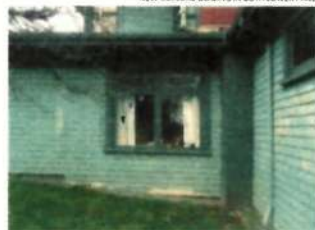
HISTORIC KITCHEN WINDOWS RESTORE WINDOW SASH TO MATCH ORIGINAL CHARACTER NEW GLASSING IN BOTH LOWER PANES
