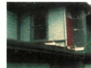
HISTORIC SITTING ROOM EXISTING DOUBLE HUNG WINDOW TO BE REMOVED AND RESTORED WITH WINDOW TYPICAL OF ORIGINAL CHARACTER WINDOW TO MATCH OPPOSITE SIDE
