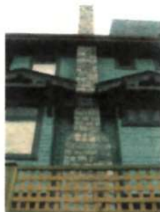
STONE CHIMNEY SERIAL RESTAINT TO BE PROVIDED STONE LINING & FOUNDATIONS TO HAVE REPAIRING AS REQUIRED
