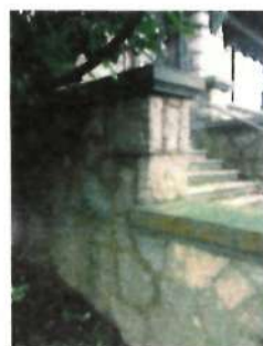
EAST WALL OF MAIN ENTRANCE STAIR STAIR PLANT WALLING IN STONE MASONRY STONE MASONRY TO BE RECONSTRUCTED & NEW SUPPORT CONSTRUCTED FROM BENEATH
