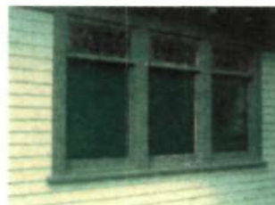
HISTORIC LIVING ROOM WINDOWS WINDOWS IN GOOD CONDITION WORK TO INCLUDE STRIPPING AND NEW PAINT
