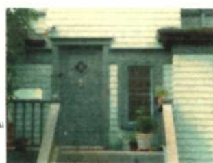
LATER ADDITION OF WINDOW (NOT ORIGINAL) FOUNDATION SAGGING ADDITION TO BE REMOVED IN ENTIRETY. WALL CLADDING TO BE RESTORED AT ORIGINAL PLANE OF EXTERIOR POTENTIAL FOR ADDITIONAL WINDOW TO MATCH ONE ABOVE OR ADJACENT
