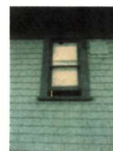
WINDOW TO BE REPLACED WITH GLASS TO SUIT NEW WINDOW GLASS TO BE REPLACED WITH GLASS TO SUIT NEW WINDOW PANEL BESIDE TO BE REMOVED AND SHINGLES TO BE RESTORED
