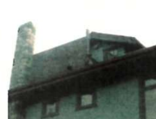
UPPER MAIN ROOF GABLE AND PREVIOUS STAIR ENTRANCE PATIOS TO BE REMOVED AND ROOF RESTORED WITH NEW SHINGLES
