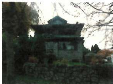
EXISTING ELEVATION SHOWING GRANITE STONE FOUNDATIONS & PILLARS
