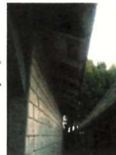
PHOTOGRAPH OF TEA HOUSE (CURRENTLY WEST) EXPOSED EAVE TO BE MAINTAINED WITH NEW PAINT SHINGLES TO BE MAINTAINED WITH STRIPPING AND NEW PAINT
