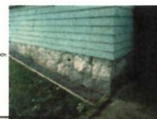
STONE FOUNDATION IN GOOD CONDITION REPOINTING AS REQUIRED
