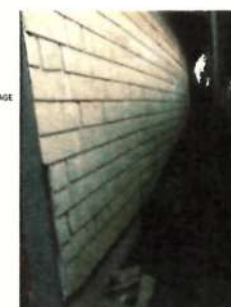
PHOTOGRAPH OF TEA HOUSE (CURRENTLY WEST) EXPOSED EAVE TO BE MAINTAINED WITH NEW PAINT SHINGLES TO BE MAINTAINED WITH STRIPPING AND NEW PAINT
