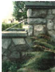
WEST WALL OF MAIN ENTRANCE STAIRS SIGNIFICANT CRACKING IN STONE MASONRY STONE MASONRY TO BE RECONSTRUCTED & NEW SUPPORT CONSTRUCTED FROM BENEATH PAINT TO BE REMOVED FROM STONE & BRICK ENTRY PORCHES & CAPS OVER STONE CAPS TO REMAIN UNPAINTED
