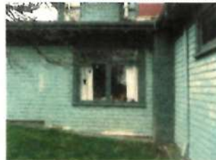
HISTORIC KITCHEN WINDOW LEADED GLASS IN GOOD CONDITION WINDOW SAGGING SIGNIFICANTLY TO THE NORTH STRUCTURAL REVIEW AND STRENGTHENING TO BE REQUIRED
