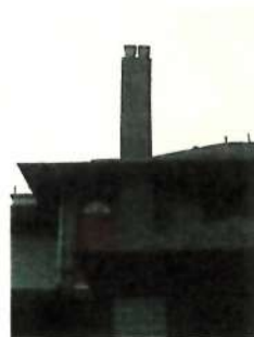
BRICK CHIMNEY (NOT ORIGINAL) CHIMNEY TO BE REMOVED AND RECONSTRUCTED IN STONE TYPICAL OF ORIGINAL CHARACTER
