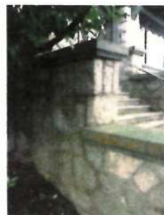
EAST WALL OF MAIN ENTRANCE STAIRS CRACKING IN STONE MASONRY STONE MASONRY TO BE RECONSTRUCTED & NEW SUPPORT CONSTRUCTED FROM BENEATH
