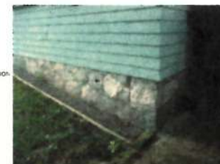
STONE FOUNDATION IN GOOD CONDITION REPAIRS AS REQUIRED
