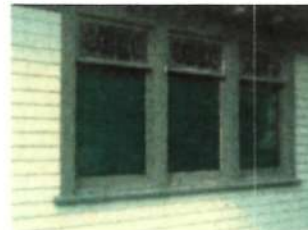
HISTORIC DEN WINDOW WINDOWS IN GOOD CONDITION WORK TO INCLUDE CLEANING AND NEW PAINT
