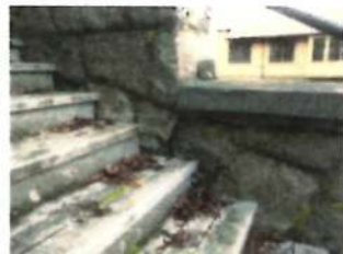
WEST WALL OF MAIN ENTRANCE STAIRS SIGNIFICANT CRACKING IN STONE MASONRY STONE MASONRY TO BE RECONSTRUCTED & NEW SUPPORT CONSTRUCTED FROM BENEATH PAINT TO BE REMOVED FROM STONE & BRICK ENTRY PORCHES & CAPS OVER STONE CAPS TO REMAIN UNPAINTED
